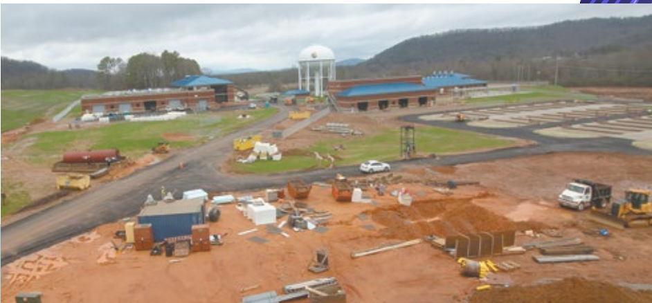
Pictured is the construction site of the new Southeast Water Treatment Plant. From June 2015 to December 2016, significant progress can be seen. The plant will add 24 million gallons a day, with capacity to expand to 96 million gallons per day.
